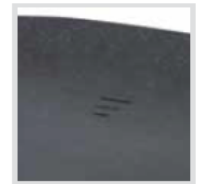
Holes for water-drainage
